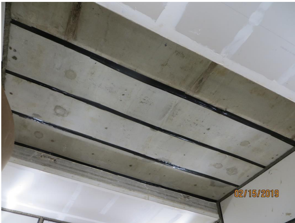
Figure 2 – Completed specimen mounted in test aperture, as viewed from receive room.
