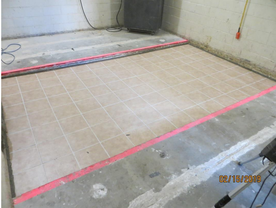
Figure 1 – Completed specimen mounted in test aperture, as viewed from source room.
