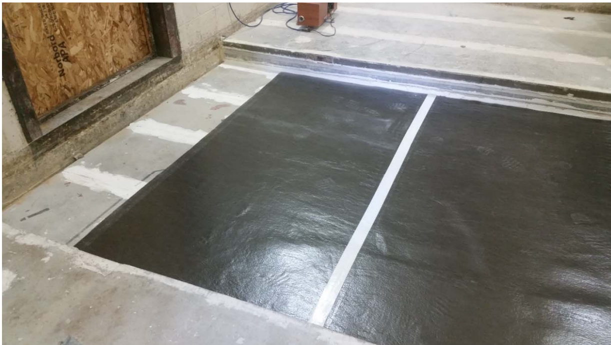
Figure 2 – Underlayment partially installed on concrete slab
