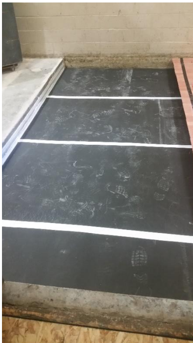
Figure 2 – Underlayment installed over concrete slab
